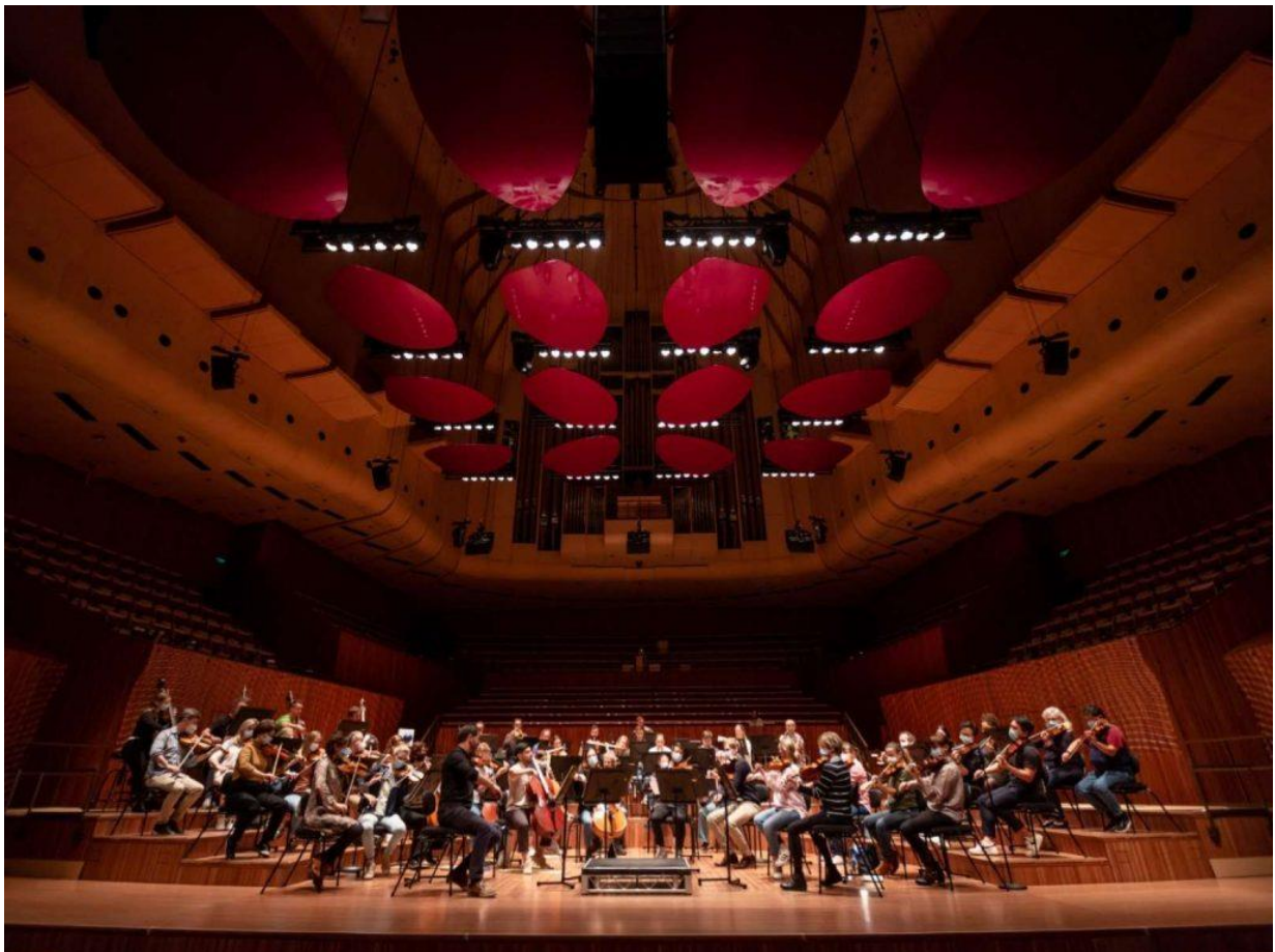
Figure 99: Sydney Opera House – Concert Hall stage with new overhead reflectors (Photography: Daniel Boud 13 )
