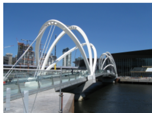
Figure 1- View of Completed Bridge
